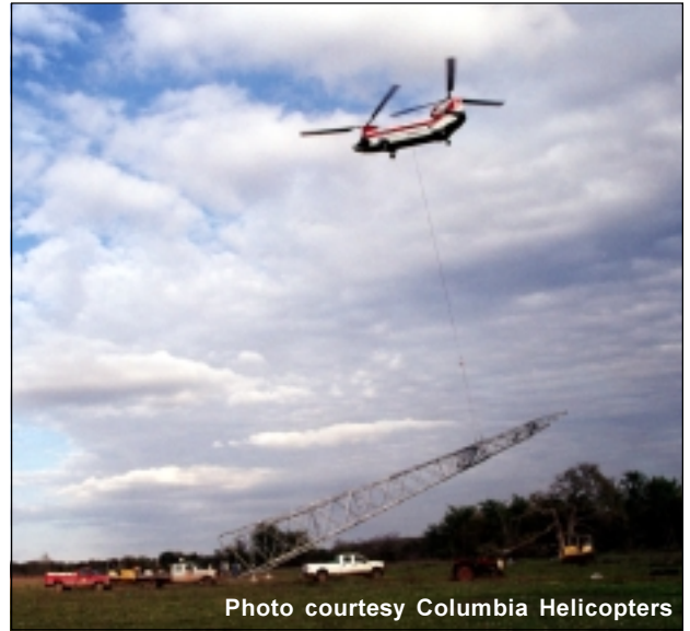
A Columbia Helicopter Chinook lifts a tower during construction.
